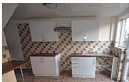
UPVC ceiling, tiled skirting and tiled instead of vinyl flooring
